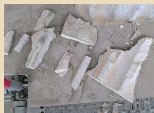
↑ Éléments de cannelure en attente de repose Fluting ready for fitting
