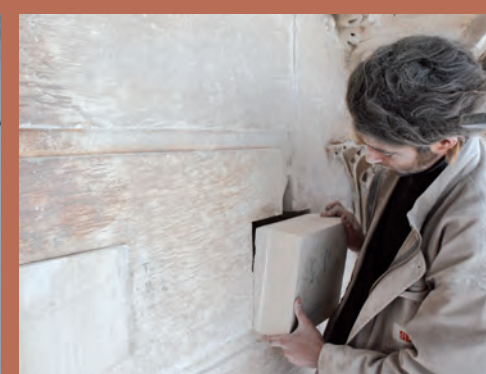
↑ Pose d'un bouchon Fitting a small graft
